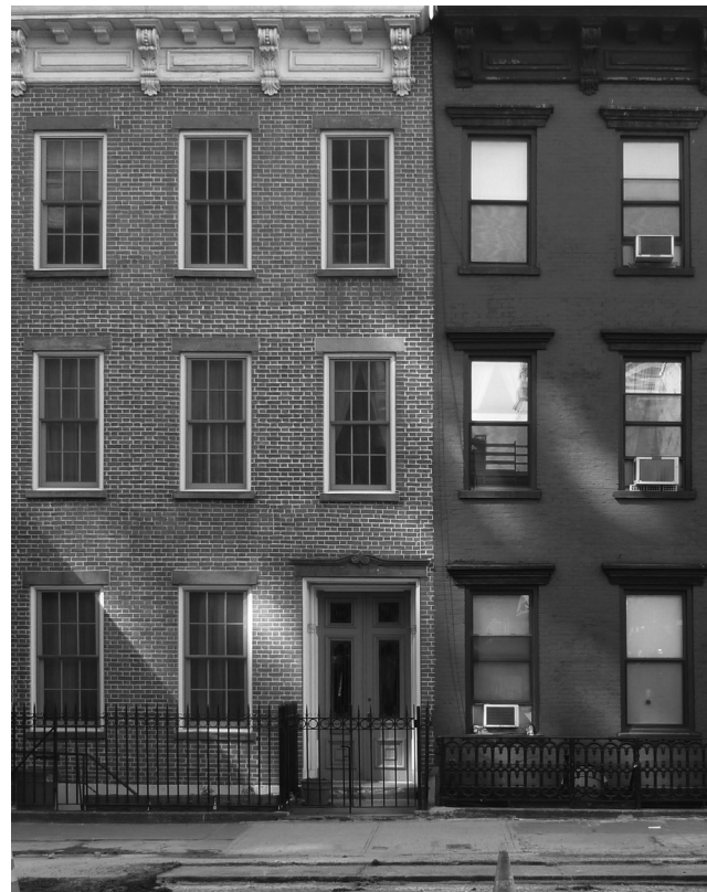
Newly designated landmarks in Community District MN02 (Greenwich Village/SoHo).
